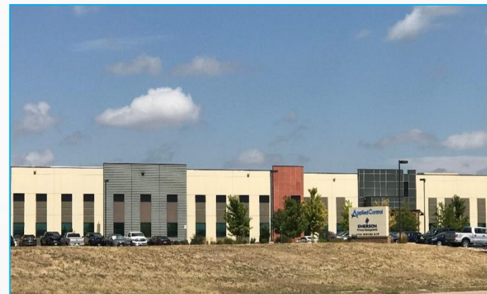
Applied Control Equipment – Denver, CO
